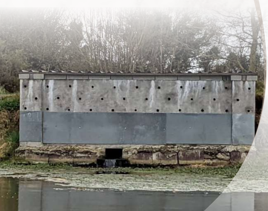
Original wall built in 2019 with the sheets of steel in place under nest entrances
